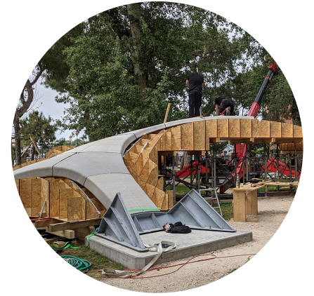
Foundations with concrete base and metal panels
