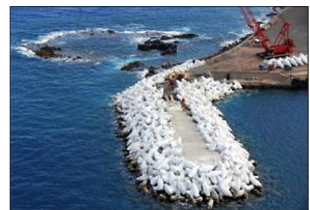
Figure 12: Kaumalapau breakwater (USACE, 2018)
