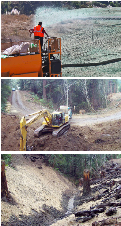
fig. 32, 33 and 34 Seeding, closure and decommission. Source: Handbook for Forest, Ranch, and Rural Roads, 2015
