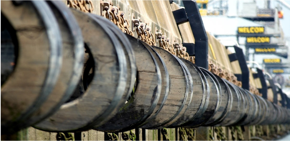
Figure 2: Cylindrical fenders at Delta Terminal Rotterdam (photo PoR)
