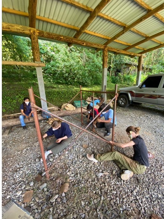
Figure 22: Sanding and painting the scaffolding (Cloud Chasers IV, 2025)
