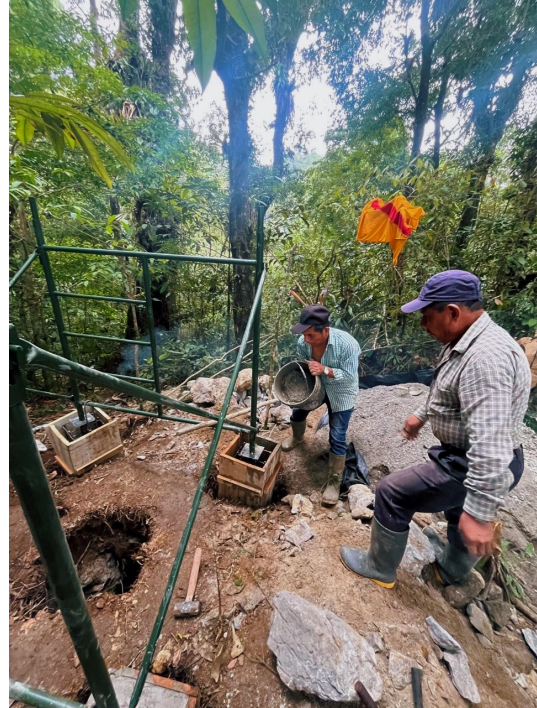
Figure 23: Pouring the concrete (Cloud Chasers IV, 2025)
