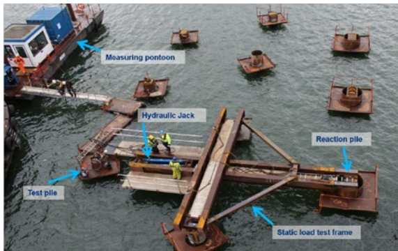
Figure 2 Overview test setup pile load test Beneluxhaven.
