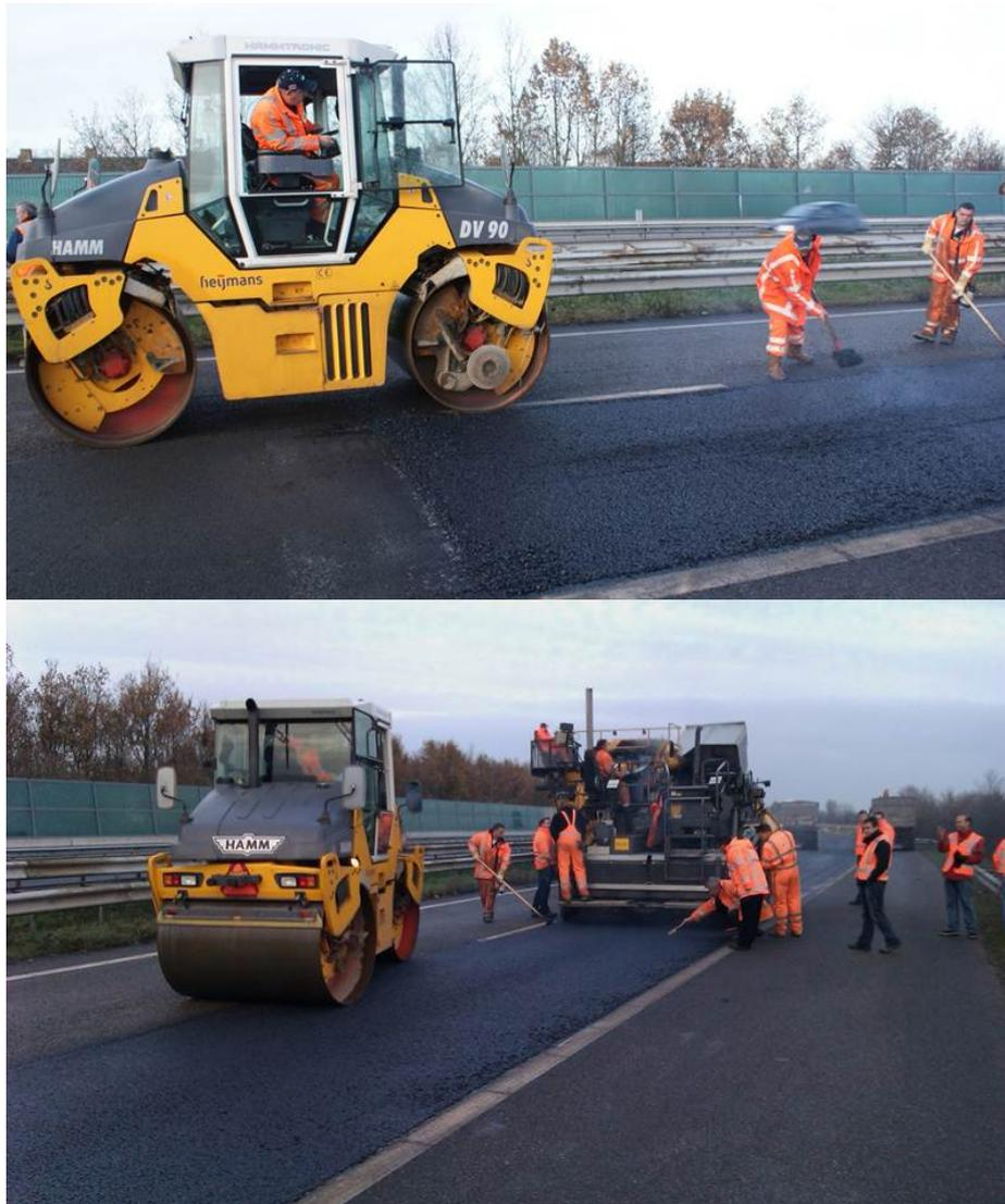
**Figure 7.11:** Construction of the induction heating trial section on Dutch motorway A58
