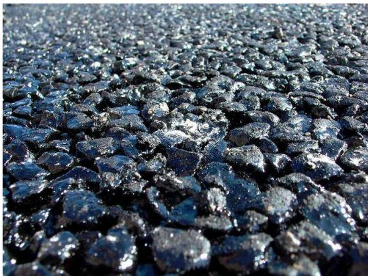
**Figure 2.3:** Standard porous asphalt 0/16 used as surface wearing course on a Dutch motorway
