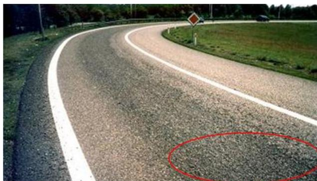
**Figure 1.1:** Ravelling in porous asphalt surface layer
