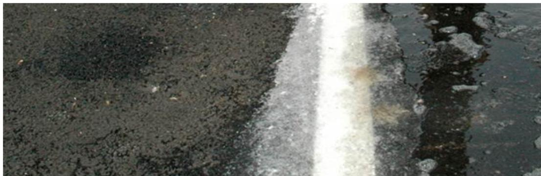
**Figure 2.4:** Comparison of a porous asphalt surface (left, clean surface) and a dense graded asphalt surface (right, wet surface with ice and water) under wet condition
