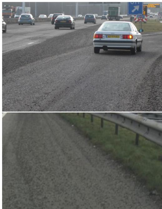
**Figure 2.5:** Serious ravelling on highways Amsterdam A1 (top) and The Hague A4 (bottom)
