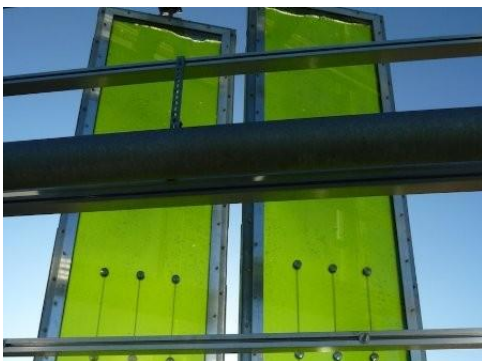
Bioreactor algae fuel façade
