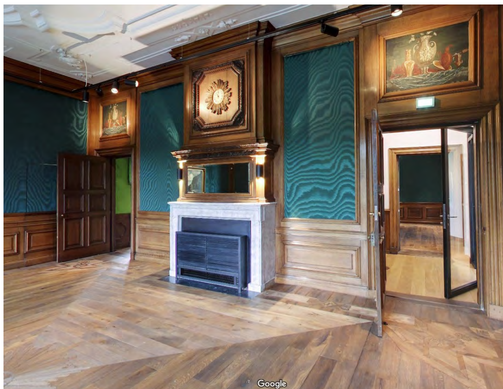
Figure 50: fan-coil unit hidden behind a grill in one of the rooms of castle Ruurlo. Image retrieved from Google Maps Streetview on May, 1, 2022.
