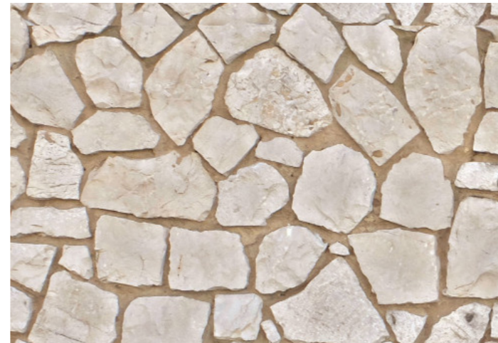
rubble stone masonry
