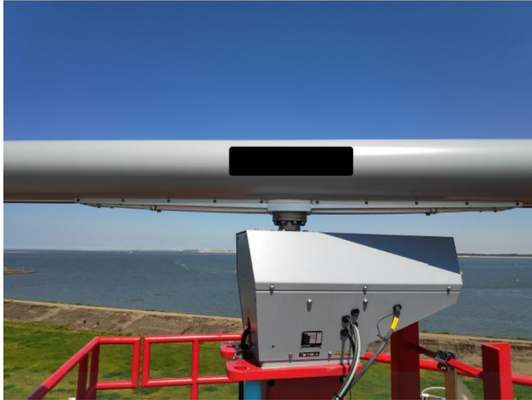
Figure 1.3.: Radar antenna and gear box on top of the mast
