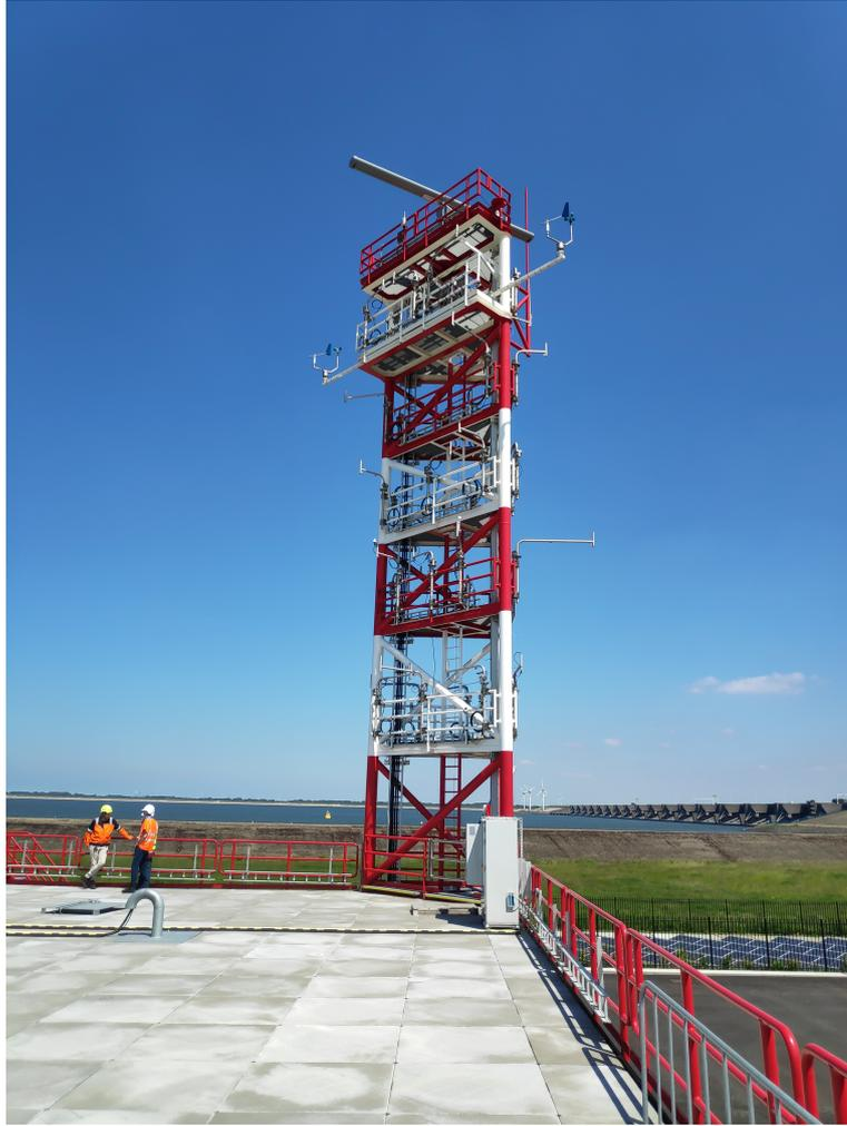
Figure 1.2.: Truss tower with the radar on top in the Offshore Expertise Center
