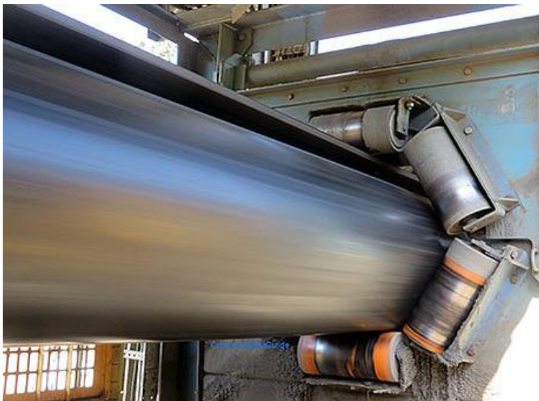
Figure 3.4: Pipe conveyor (Image courtesy of Bridgestone Corporation)
