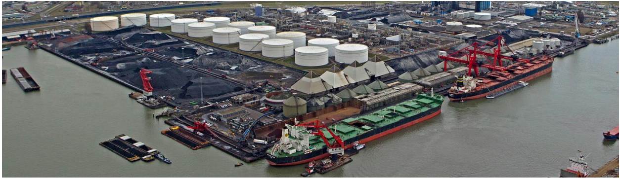
Figure 3.8: St Laurens haven terminal aerial view (Image courtesy of EBS B.V.)
