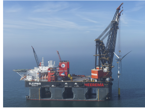
(b) Heerema's SSCV Sleipnir performing a floating installation of an offshore wind turbine [39].
