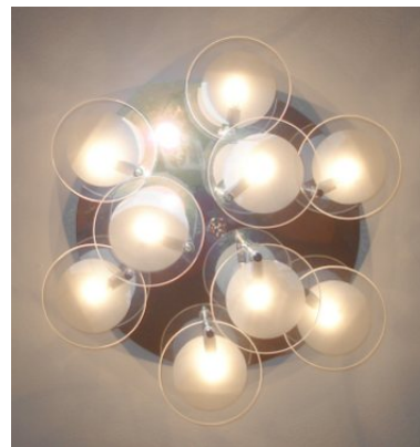
Figure 10.2 – Halogen ceiling luminaire with many 20W halogen lamps ('7 days more light', Voldersgracht, Delft).
