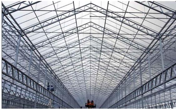
**Figure 5.5:** Example of a Widespan greenhouse system, image provided by Boal Systemen
