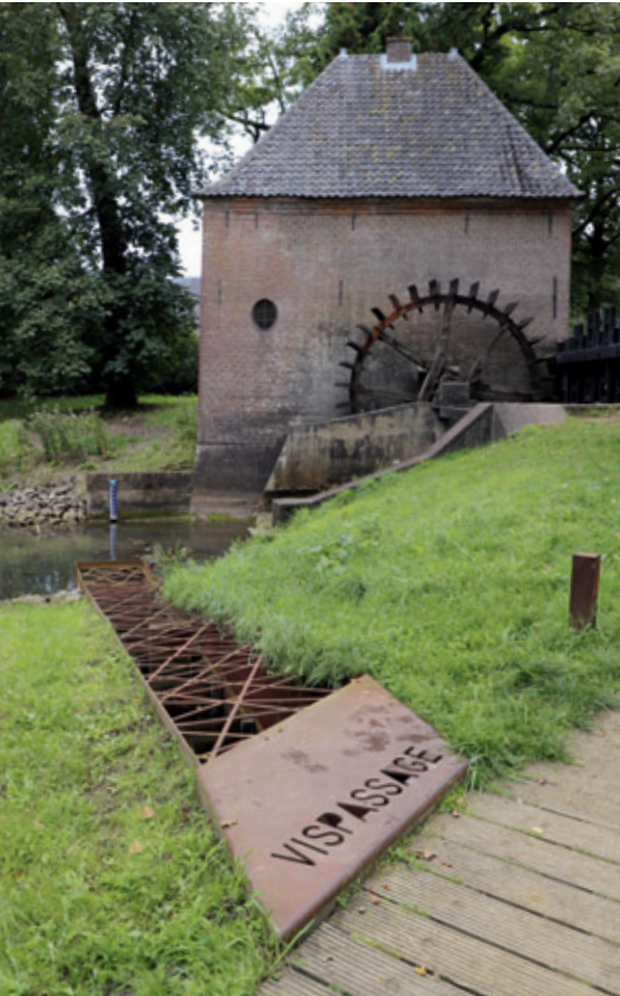
[FIG. 08] Newly added fish passage connected to the historical watermill at Hackfort. (Photo: Steffen Nijhuis, TU Delft)
