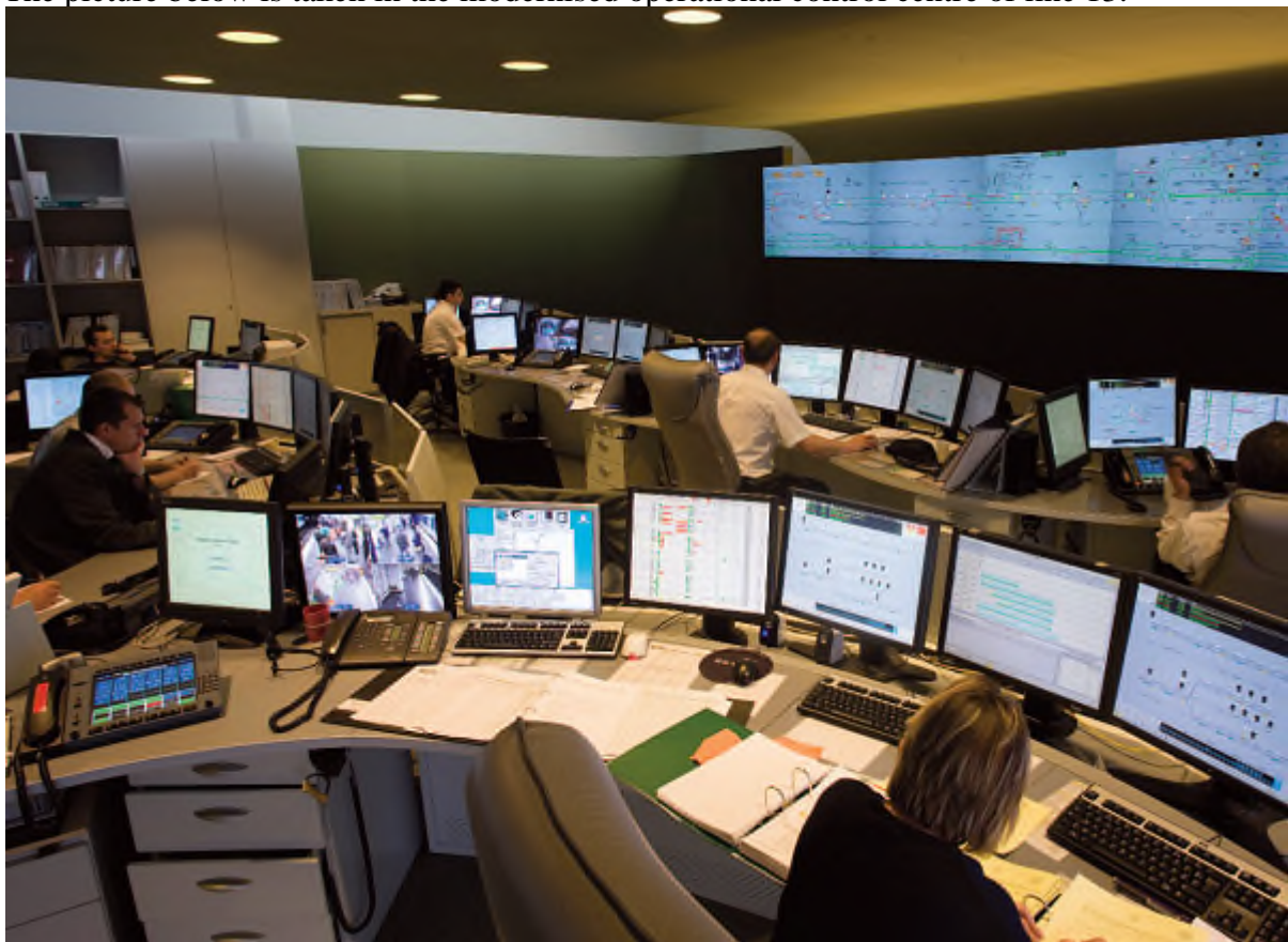
Figure 18 – Inside the modernised operational control centre (PCC) of line 13
