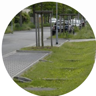
Figure 2. Disconnect rainwater (visibly) 3
