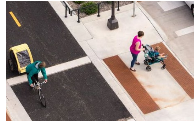
Inclusive streets with safe crossing spots with ridges that can be felt for vision problems
