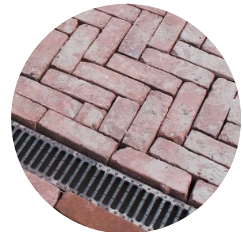
Figure 9. Use of water gutter in the areas of surfacing 9
