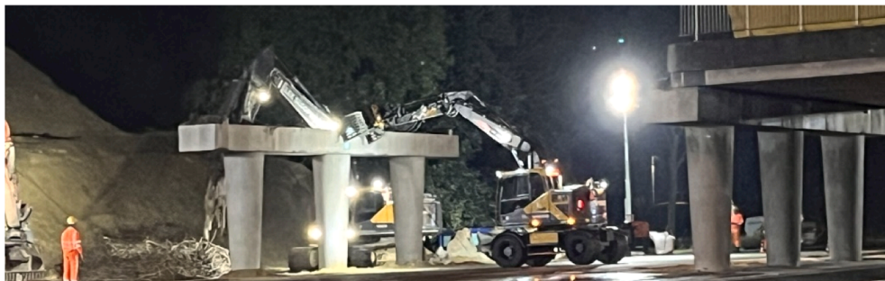
f) Simultaneous demolition of support beams and columns.
