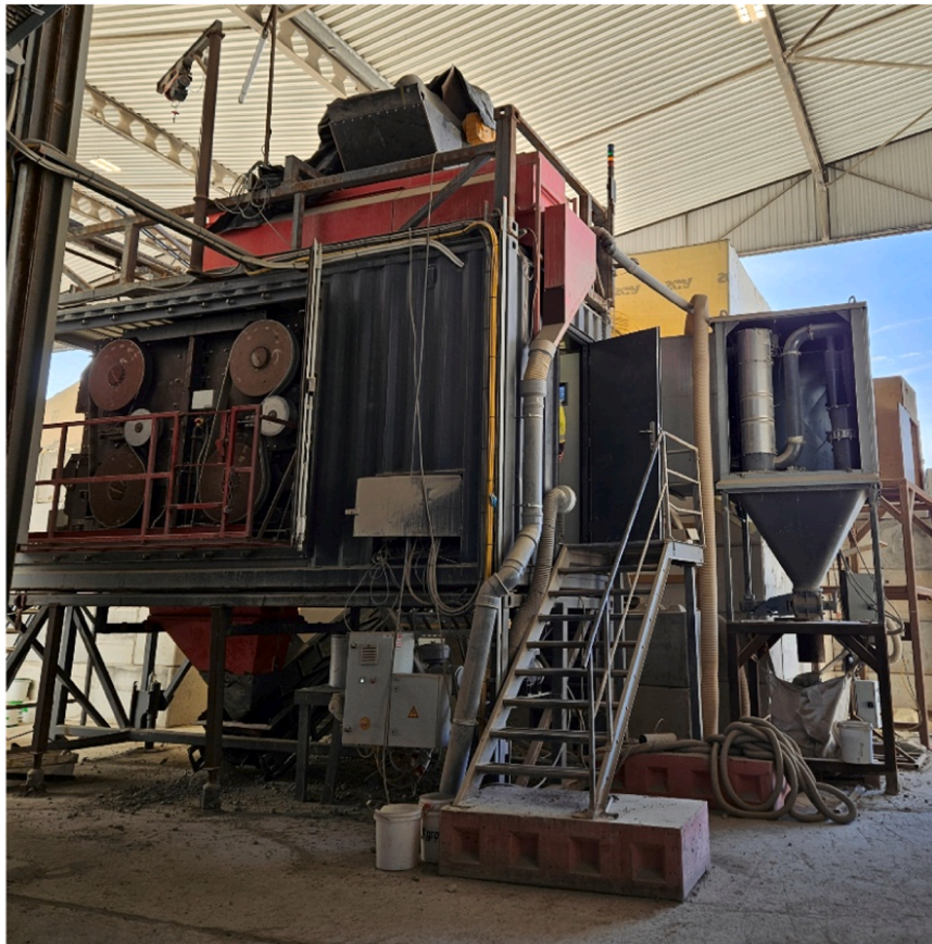
Fig. 3. Smart Liberator, industrial-scale recycling technique for concrete.
