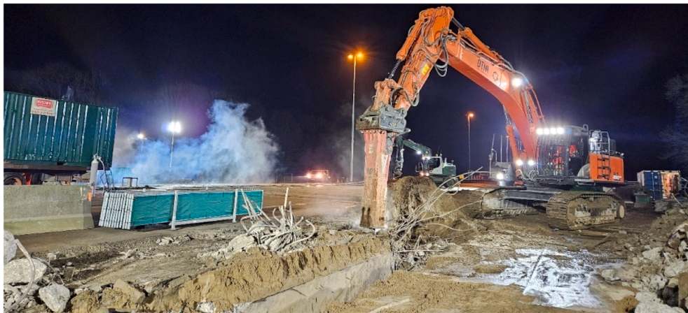
g) Demolition of the foundation.
