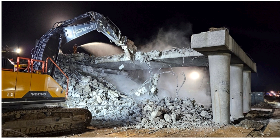
e) Demolition of deck 1 (T-beams).
