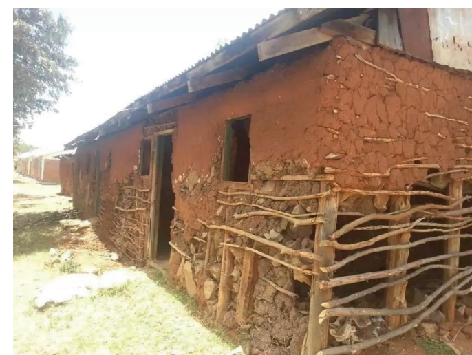
Figure 29. Mud wall with crack
