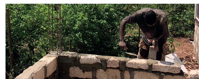
Figure 27. Masonry fundi laying coral blocks
