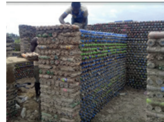
Figure 41. Plastic bottle structure in Nigeria (Oyinola et al., 2018)
