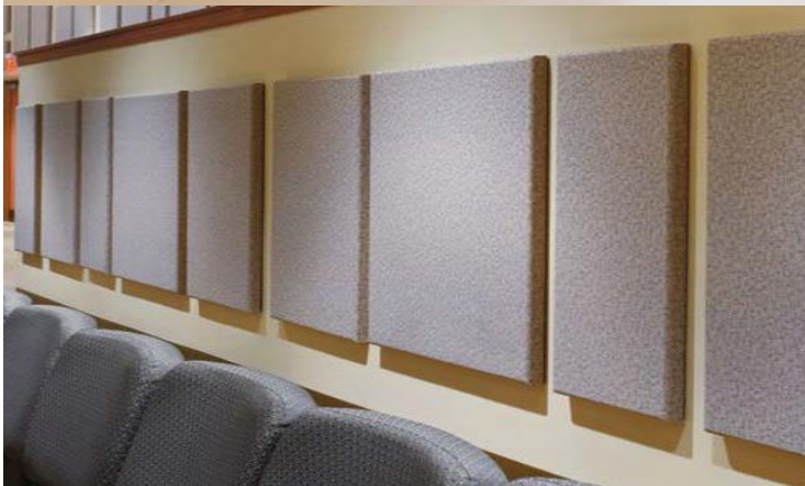
Figure 44: Existing acoustic wall covering
