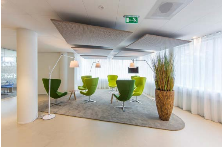
Figure 43: Existing suspended acoustic panels
