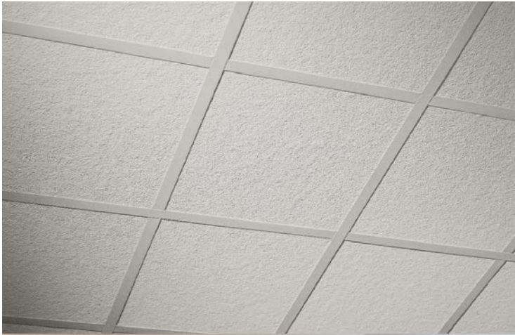
Figure 42: Existing ceiling tiles
