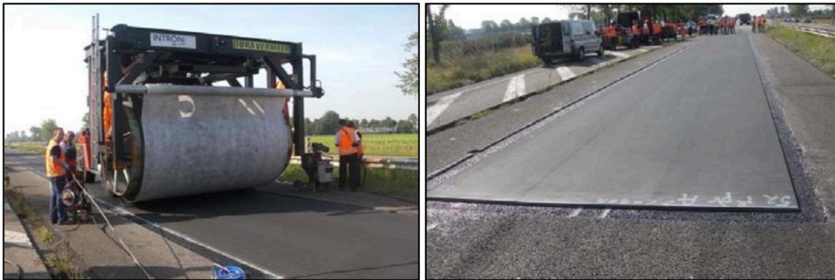
Figure 2.2: Application of PERS on the A50 near service area De Brink using the Rollpave technique [10]
