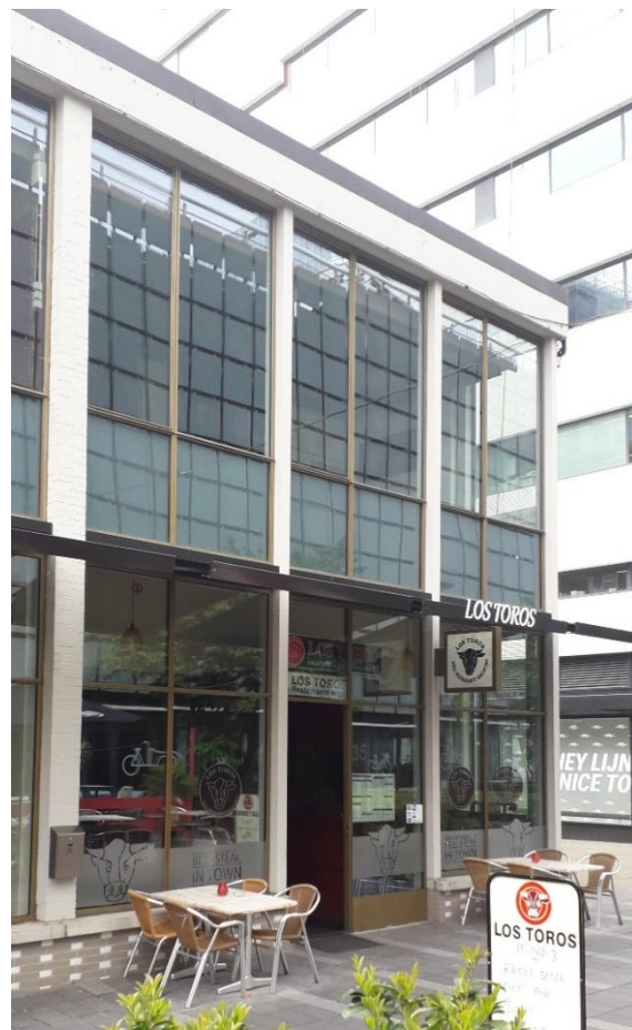
Fig.7: Photograph of one of the shop facades after the renovation. Note the brick bond near the base of the façade, the brass profiles in the glass façade and the lack of wooden canopy. A.Dolieslager, 2023.
