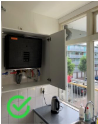
Figure 12: Approved location: HIU placed in a kitchen drawer (image retrieved from the energy company).
