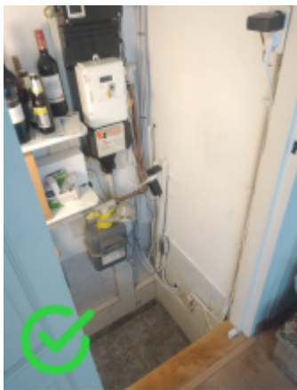
Figure 13: Approved location: the meter cupboard (image retrieved from the energy company).
