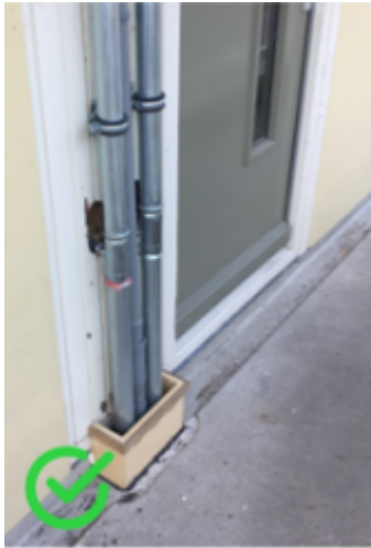
Figure 15: Approved locations: risers through the gallery (image retrieved from the energy company).
