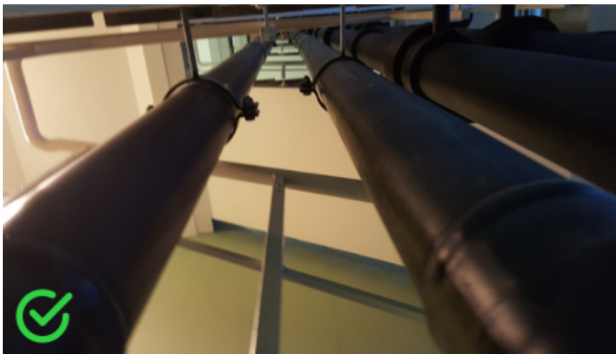
Figure 16: Approved locations: risers through the stairwell (image retrieved from the energy company).
