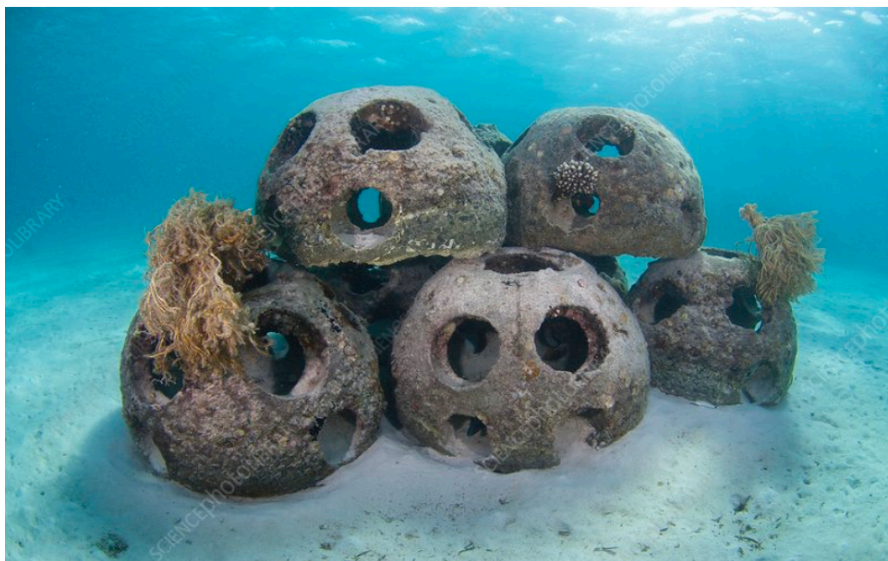
Figure 4.4: Example of deployed Reef Balls used for marine habitat restoration. The hollow, perforated design enhances hydrodynamic stability and provides complex habitats for colonization [Reef Ball Foundation, 2025].
