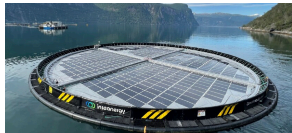
(b) Circular floating solar array co-located with aquaculture cages (Inseanergy pilot, Norway) [Santos, 2023; Team, 2022].
