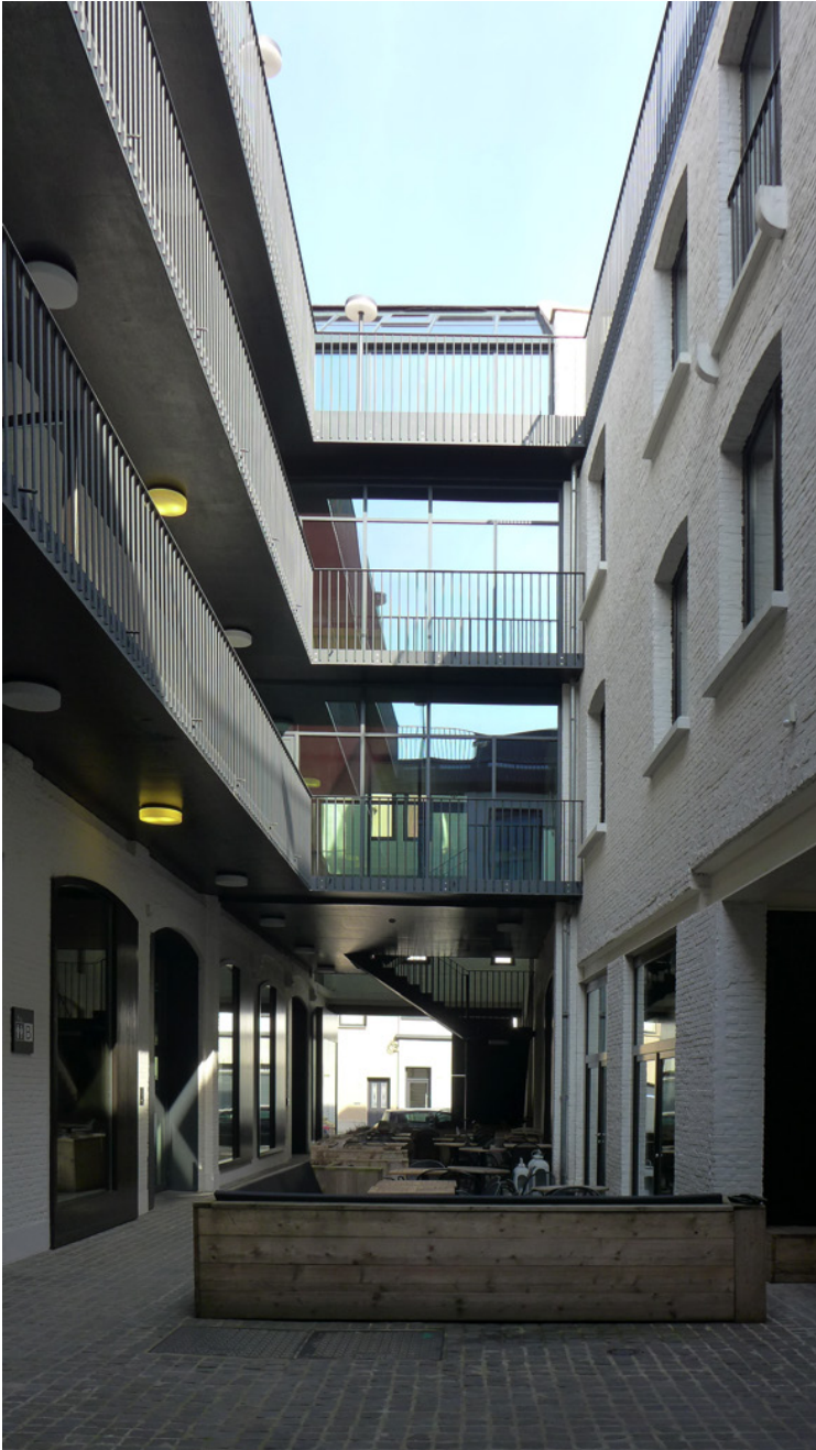
FIGURE 5 Inner street of the Valkeniersnatie was made public by architects Robbrecht and Daem. Spaces for restaurants and shops are foreseen on ground level.
