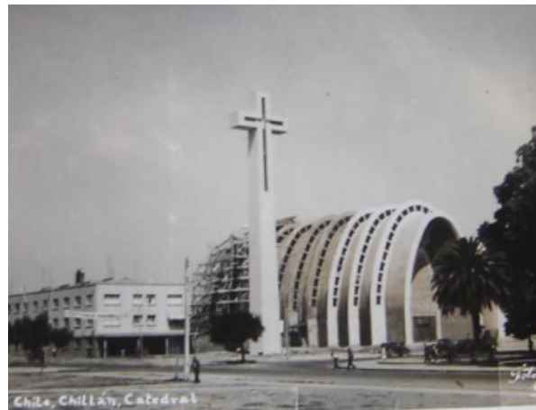
FIGURE 5 Chillán Cathedral and Plaza after reconstruction
