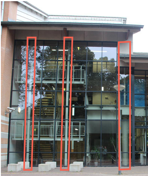
Image 65 Steel columns glass facade
