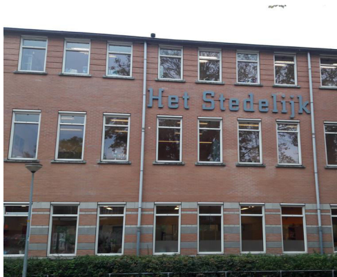
Image 75 Front facade A and B
