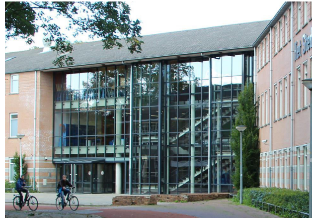
Image 80 Glass facade between A and B
