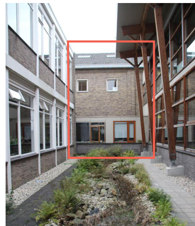
Image 53 North inner facade
