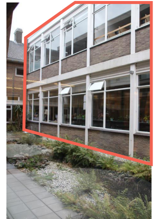
Image 52 West inner facade
