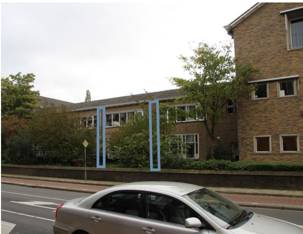
Image 60 brickwork pillars non constructive
