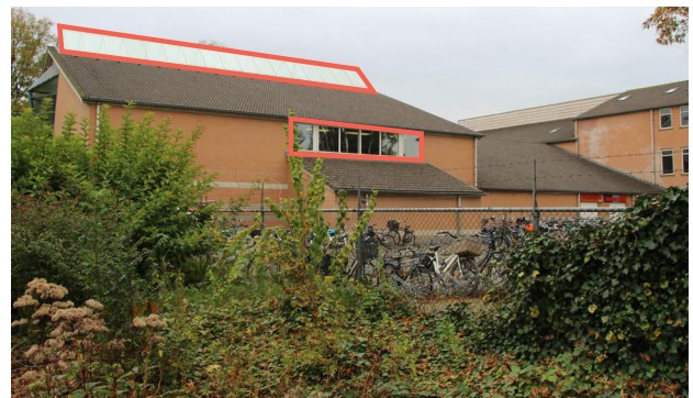
Image 82 West facade gym
