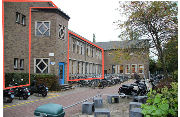
Image 59 bearing facade with big openings
