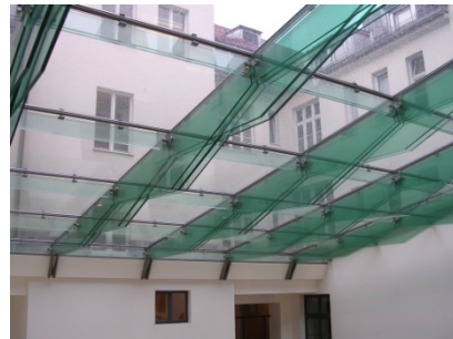
Figure 2.5: Segmented 14 m glass beams applied in the atrium roof covering of the Industrie Handelskammer building in Munich, Germany [Betsch, 2004].
