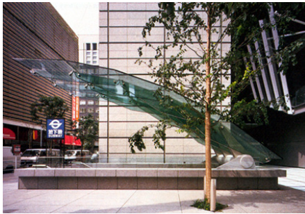
Figure 2.4: Segmented 9 m glass beams applied in the Yurakucho metro station entrance covering, Japan; Engineer: Dewhurst Macfarlane
