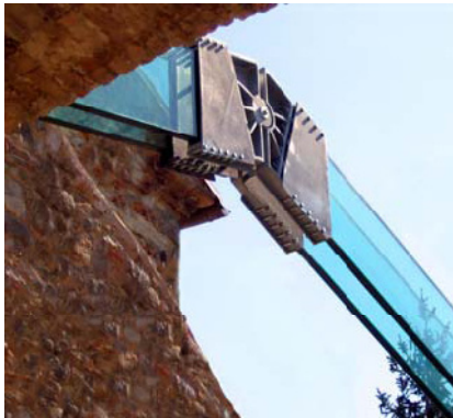
Figure 3.22: CFRP reinforced glass beams [Palumbo, Palumbo & Mazuchelli, 2005].
