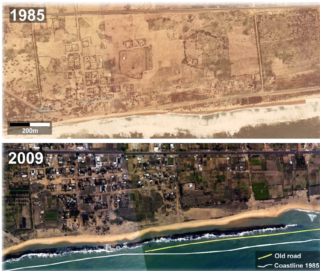
Figure 15 Coastal evolution at PK20 1985-2009: Appearance of beachrock, destruction of old road and increased population pressure. Images courtesy CGILE
