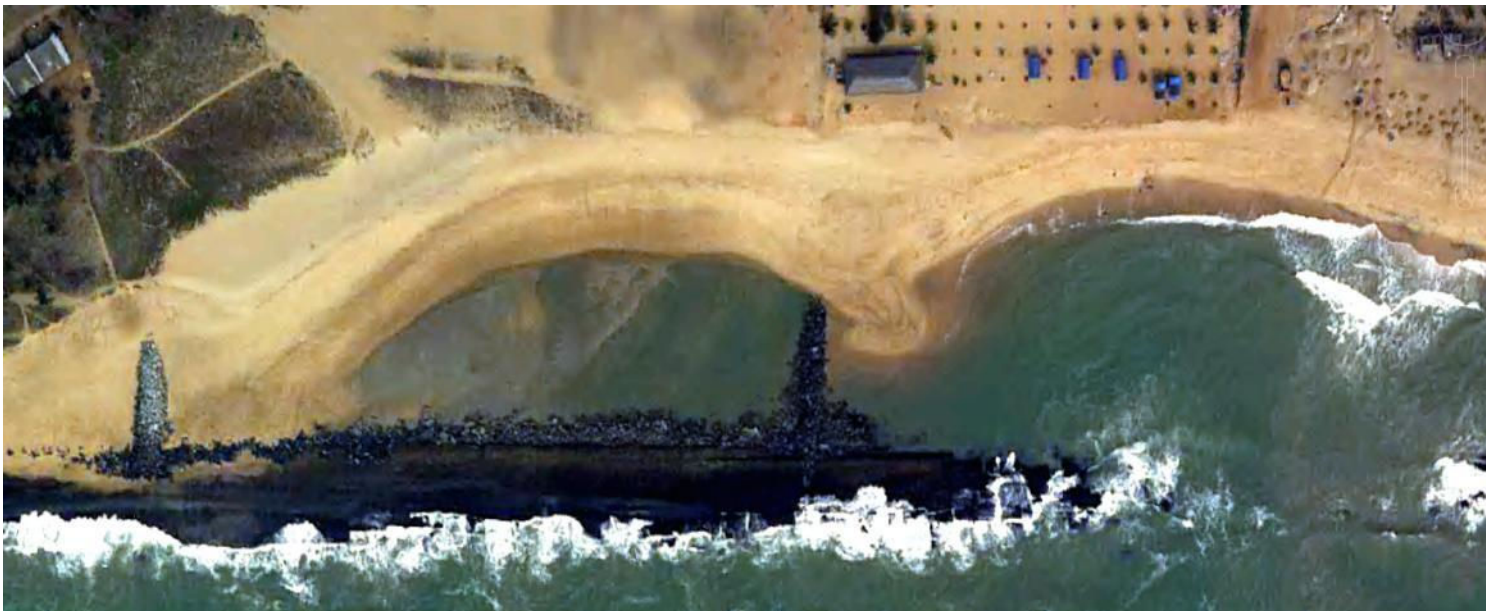
Figure 5 Transect #3 Detail B: Engineered structures
