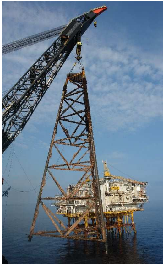
Figure 12: Jacket removal
