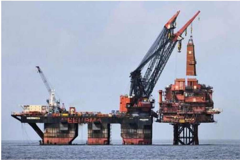
Figure 7: Drilling tower removal (Berghuis)
