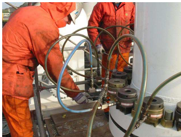
Figure 72: Hydraulic bolt pre-tensioning
