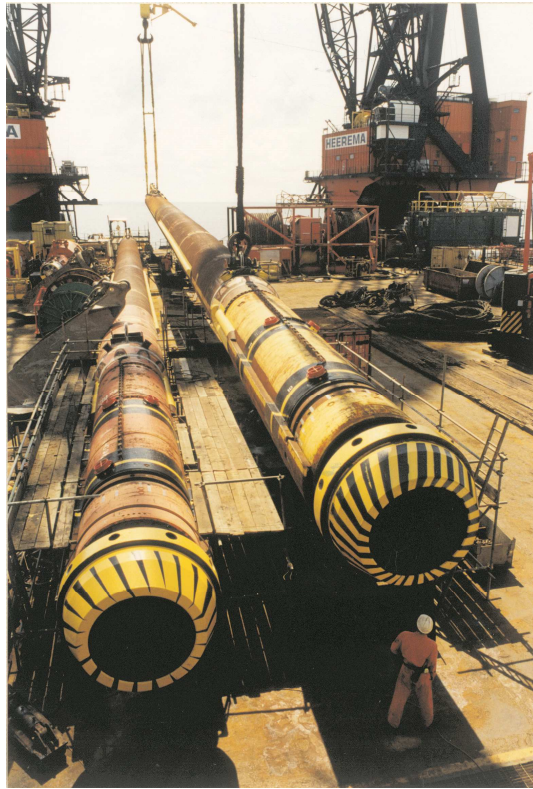
Figure 43: Upending of piles (HMC)
