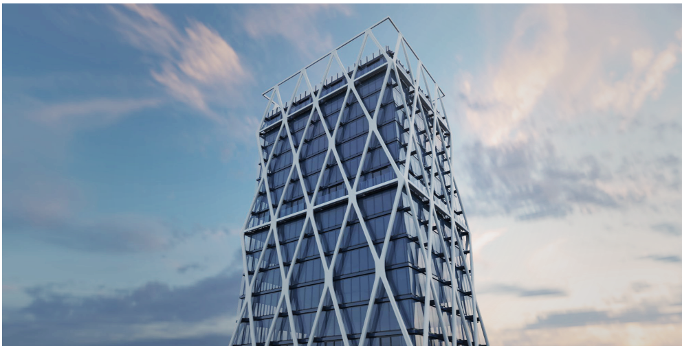
Figure 41: Top levels of the building
