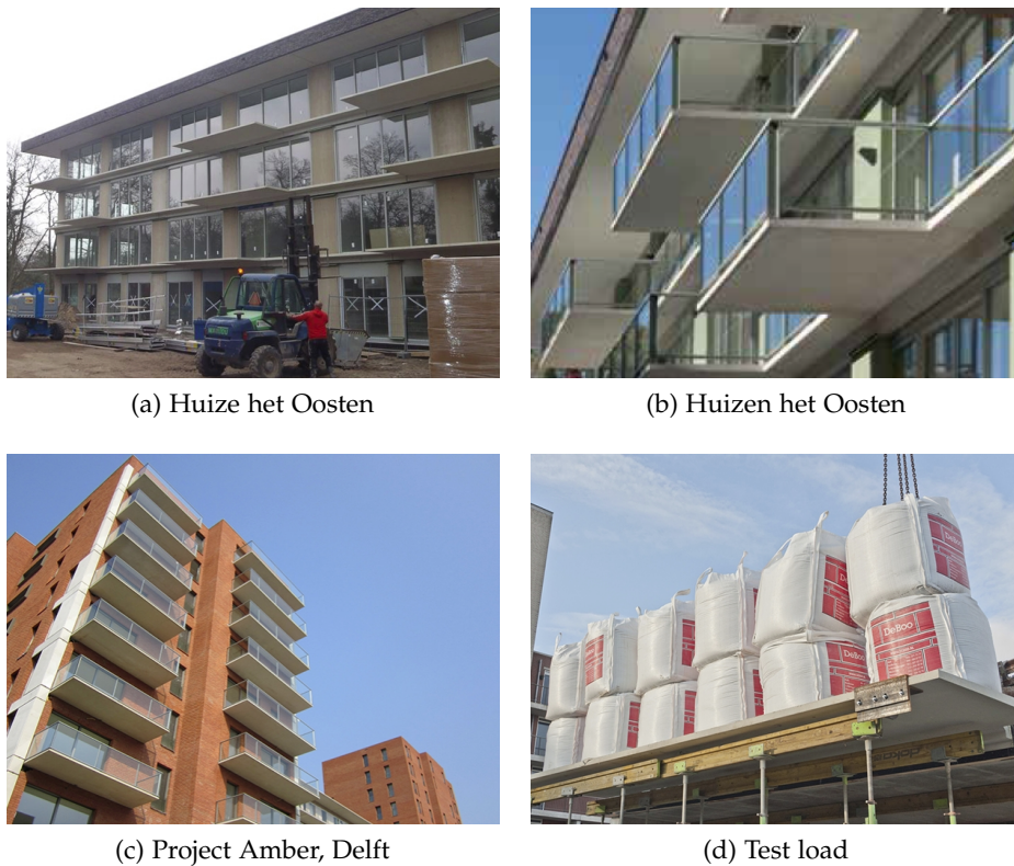
Figure 6: Huize het Oosten [50], UHPFRC used for ultra thin balconies for residential buildings
