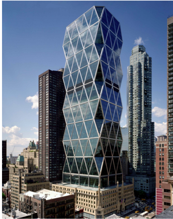
Figure 13: Hearts Tower in New York by Foster + Partners, [51]
