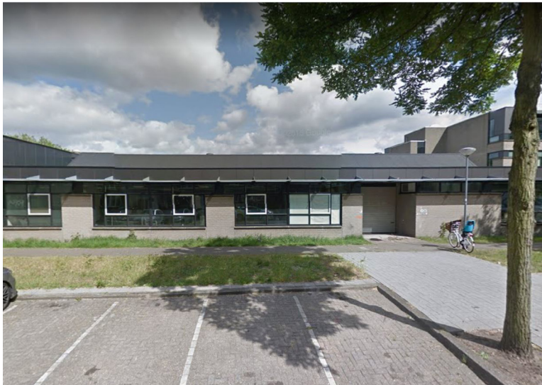
Figure 87 Location of the design intervention of patching in between the residential buildings of Schiemond and the harbour inlet. In addition, a picture of the current view once a citizen leaves the residential buildings of Schiemond. Currently a 135 meter long building is blocking the connection
