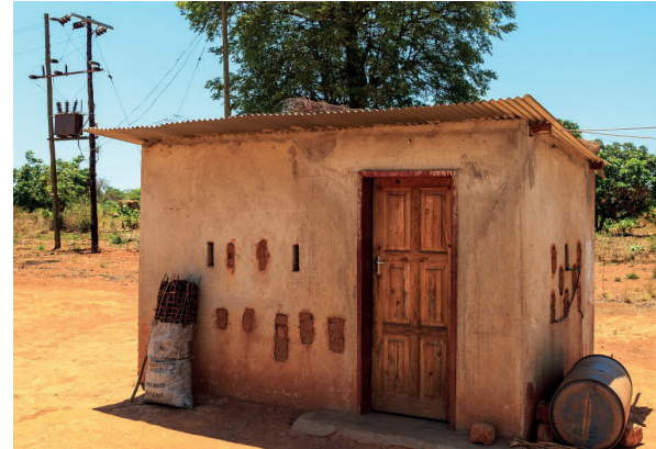
Electricity house, By: Econoler
