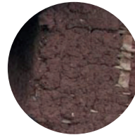
Earth filled walls
