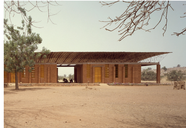
Primary School Gando (2001)
