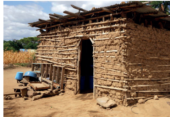
House, by: Habitat for Humanity
