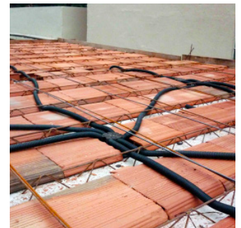
beam and block floor
