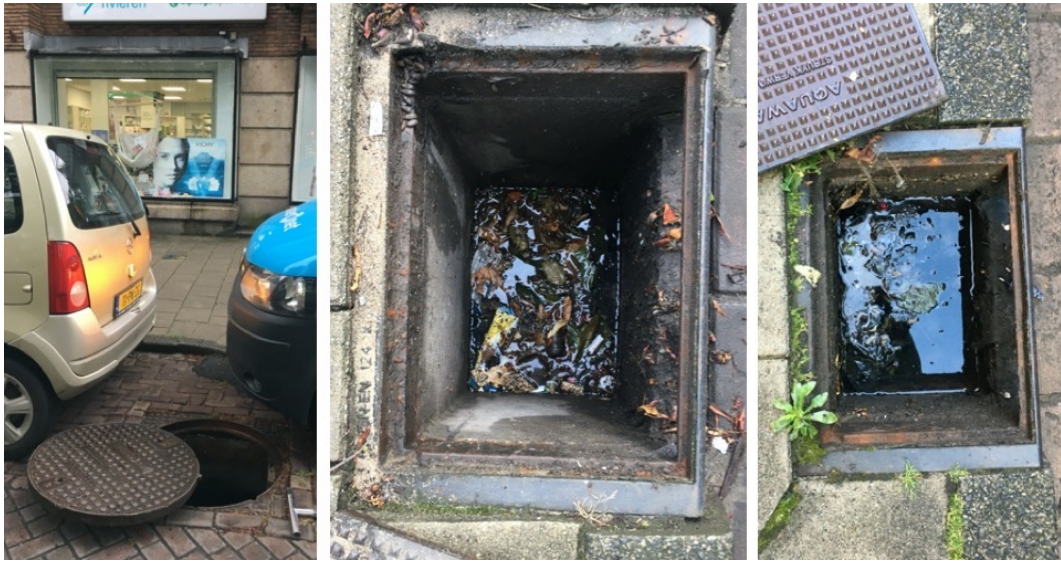
Figure D-1 left: location manhole; middle & right: location gully pot.
