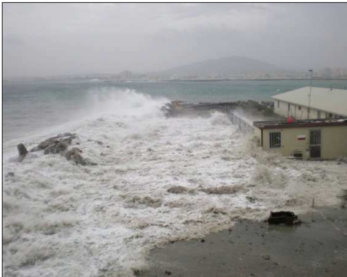
Figure 1 Damage caused by wave overtopping
