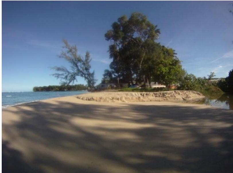
Figure 42 - Stormwater Discharge Outlet in Holetown showing the inner basin, the scour channel, and subsequent natural closure of the outlet by wave action
