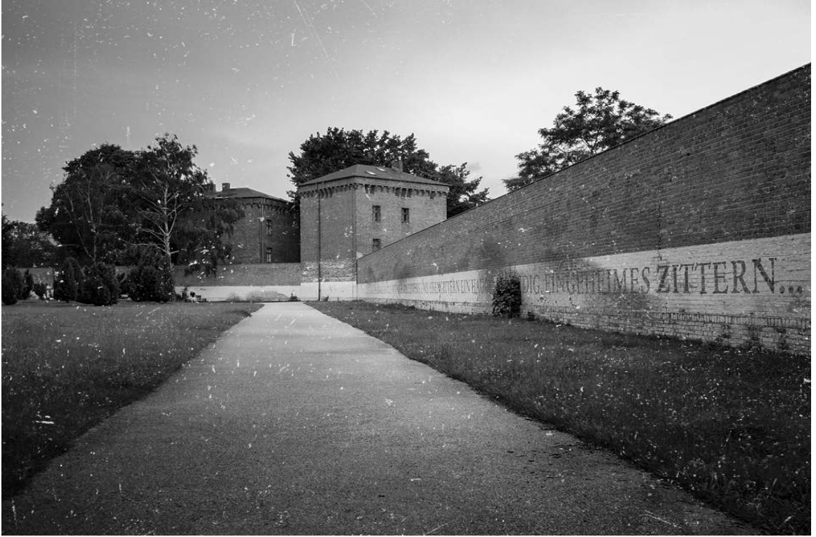
Fig - 19. Remains of the prison walls and the Guard residences.
