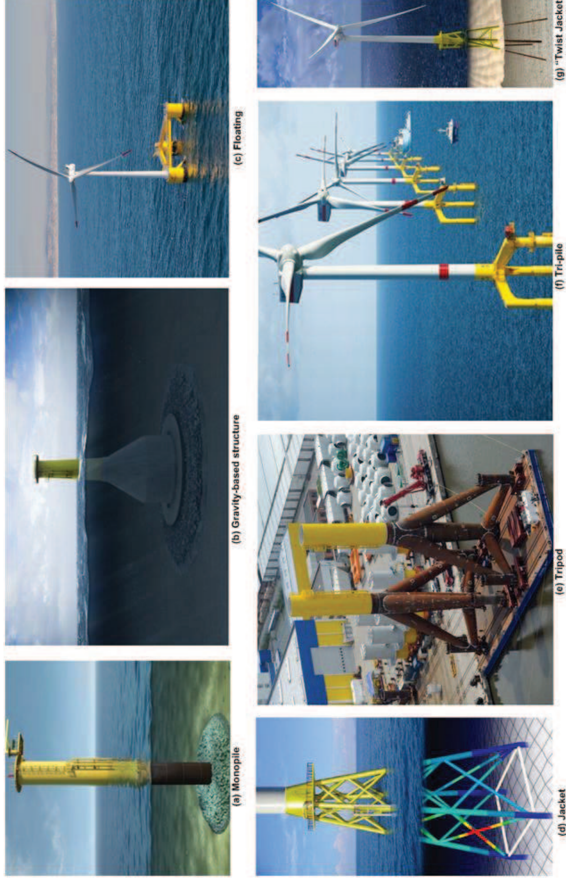
Figure 2-5: Different types of wind turbine foundation.
