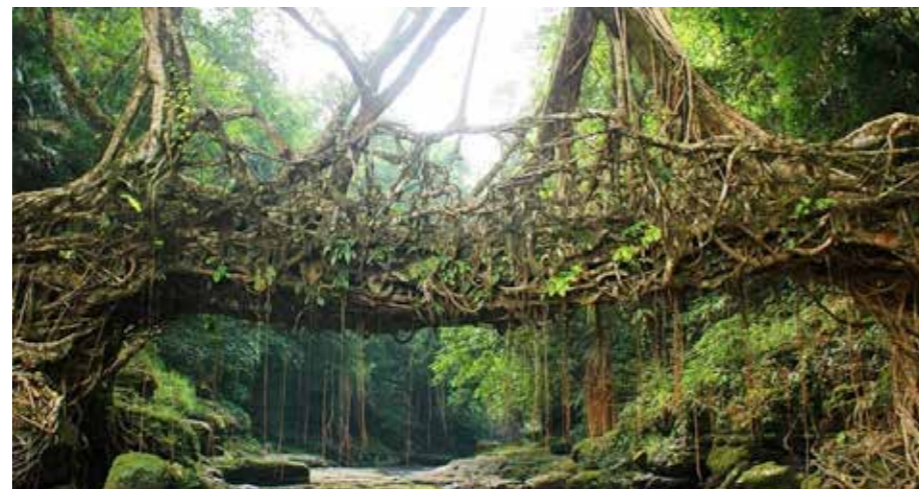
Figure 56: Living Root Bridges, Bangladesh
