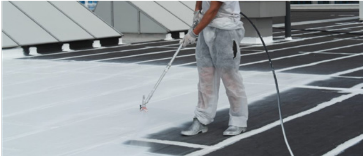
Figure 6.9 Picture of white coating being applied to a roof
