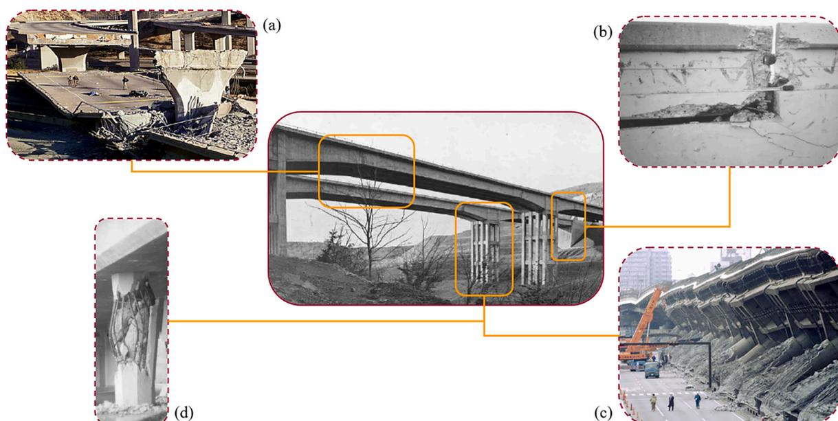
**Fig. 1.** Typical damages in the bridge structural components during an earthquake. a) Deck unseating and bearings failure (Northridge 1994); b) Pounding between deck's components (Northridge 1994); c) Columns failure (Kobe 1995); d) Column failure (San Fernando 1971).
