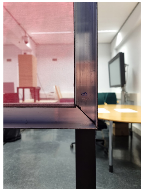
Figure 5.28: Intersecting of U-profiles
