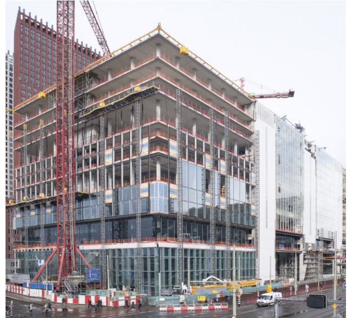
Fig. 5.3.3 Extension on the south side - prefabricated panels (Vorsselmans, n.d.).
