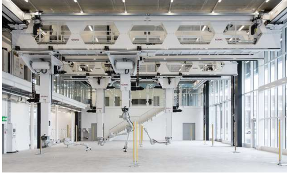
Figure 9.9: Spatial robotic assembly at ETH Zürich | ETH Zürich
