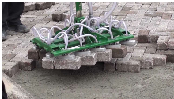
Figure 12.5: The placement of paving bricks with the help of a vacuum suction cup.
