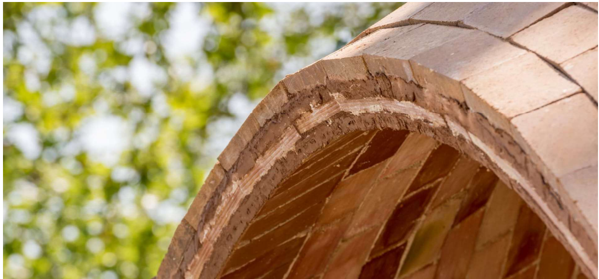
Figure 1: Example of thin-tile vaults: Droneport.
