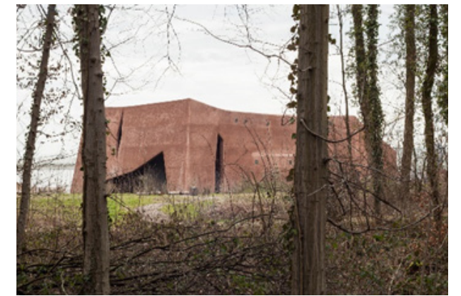
Figure 9: Muttentz Water Purification Plant in Muttentz, Switzerland by Oppenheim Architecture + Design, 2017 (Müller, 2017)
