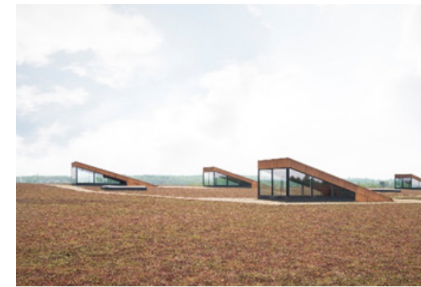
Figure 8: Solrødgård Water Treatment Plant in Hillerød, Denmark by Henning Larsen, 2017 (Due, 2017)
