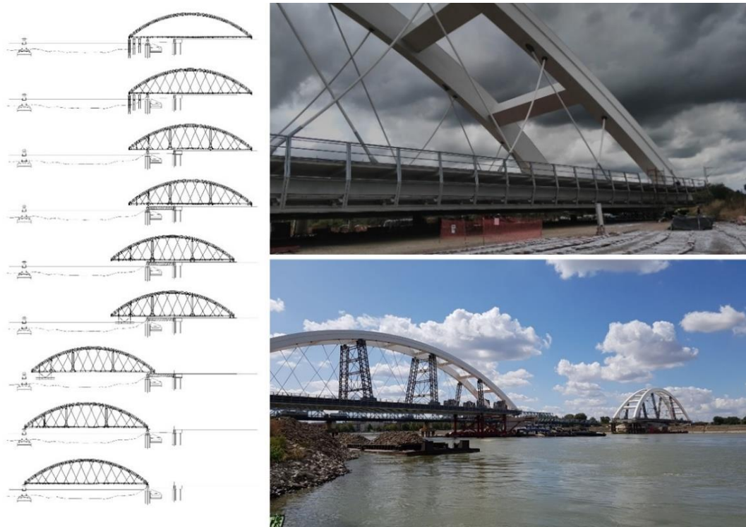
Figure 9. Launching of arch bridges over the Danube.
