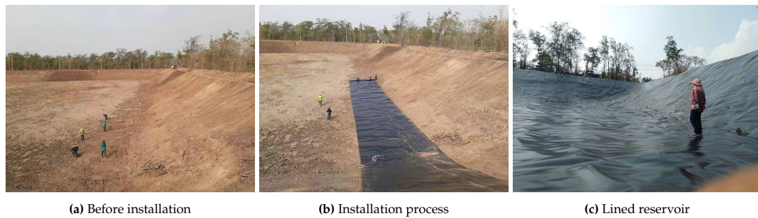
Figure 6.4: Example of geomembrane installation in a reservoir [72]
