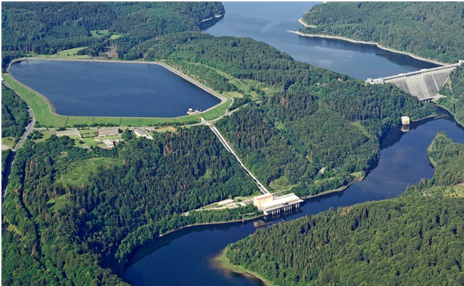
Figure 2.8: Open loop pumped hydro energy storage [45].
