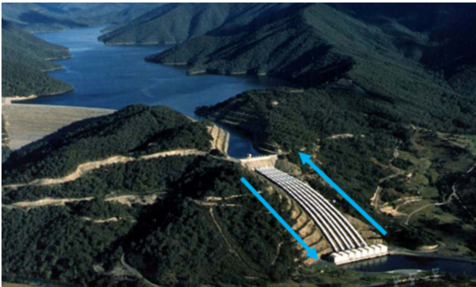
Figure 2.7: Pumped-back pumped hydro energy storage [44].
