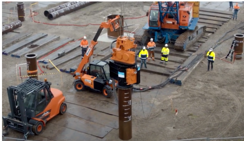
Figure 1: Medium-scale pile installation tests in an onshore sandy site.
