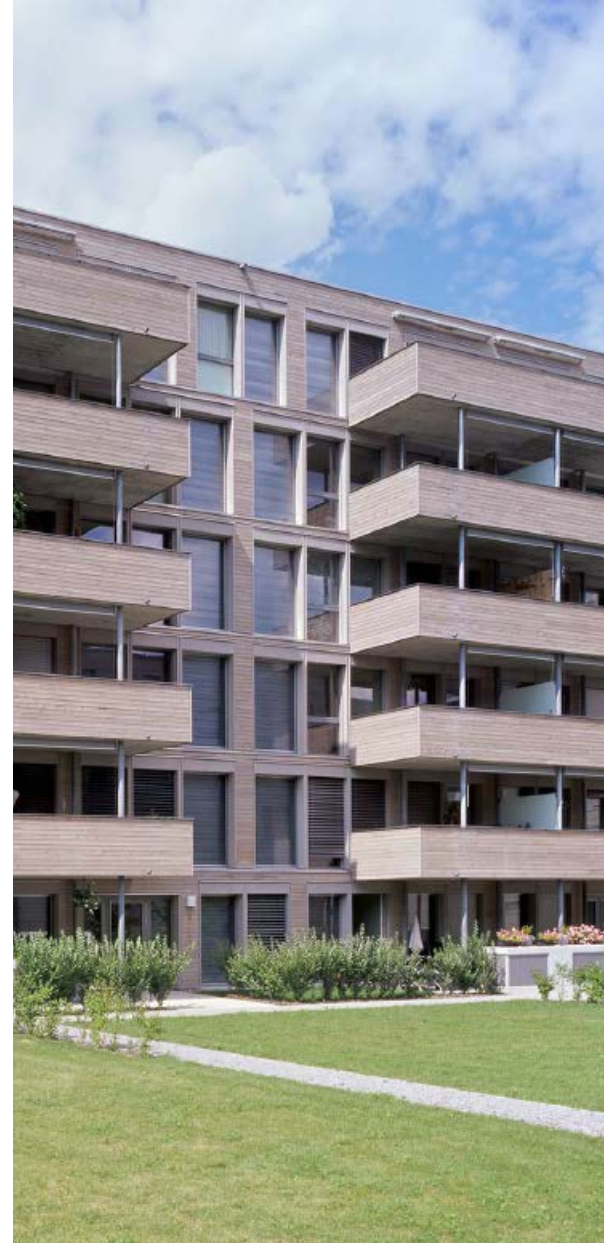
Figure 37: The facade of the Eulachof Building, integrating GlassX products, Reviewed from: http://www.schwarz-architekten.com/en/project/
