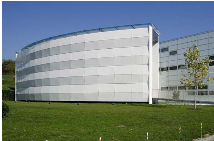
Figure 26: The facade responding different in order to provide changing shading levels, Reviewed from: http://www.dailytonic.com/dynamic-facade-kiefer-technic-showroom-by-ernst-giselbrecht-partner-at/ .
